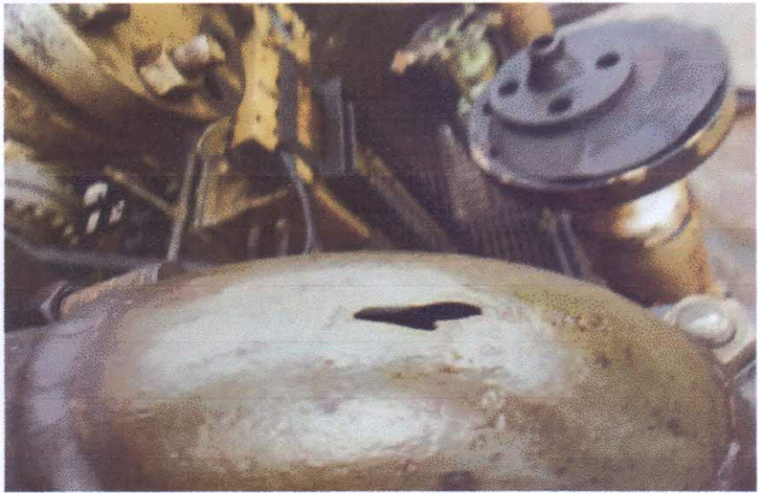
SPILL POINT: fig1
